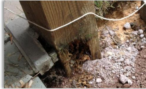
**Water Damage Deck Support on 25-30 year old Deck**
